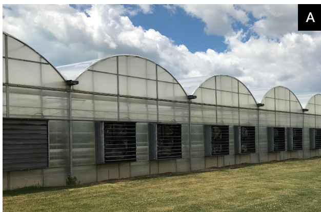
Figure 10. (A) Traditional horizontal fans on the side of a low tomato greenhouse. (B) Modern horizontal fan above a tomato crop in a tall greenhouse. (C) Modern through-curtain fan.
