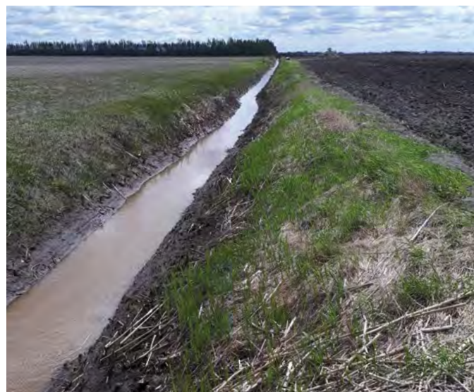
Figure A3-11. A bottom cleanout of a drain with vegetation remaining on the bank. Source: Leroux Consultant, Municipality of Alfred-Plantagenet, Ontario
