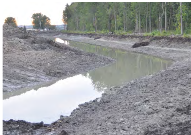
Figure B4-17. A dewatered channel with a littoral shelf on the right side of the channel.
