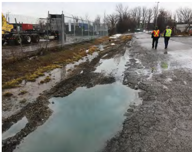
Figure B5-22. Southdown – drainage issue despite the existence of storm sewers.
