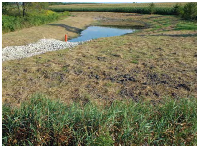
Figure B4-25. Straw/hay mulch spread on exposed soil surrounding a sediment trap. Source: Ausable Bayfield Conservation Authority, Ontario
