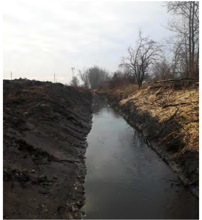
Figure A3-13. A recently completed full drain clean out. Source: Dietrich Engineering Ltd., Kitchener, Ontario
