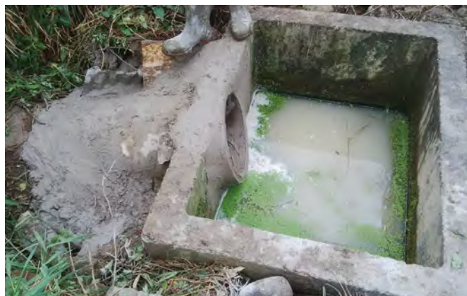
Figure A3-14. Repairs being made to a junction box. Source: Dietrich Engineering Ltd., Kitchener, Ontario
