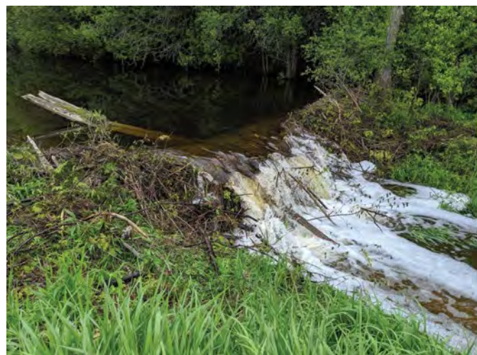
Figure A3-5. A beaver dam obstructing the flow of a drain. Source: City of Kawartha Lakes, Ontario
