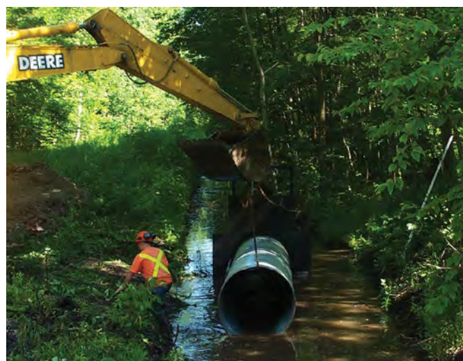
Figure B5-16. Dry Creek – installation of one of the water control structures.
