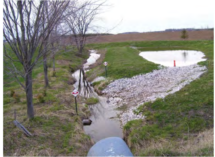
Figure B5-7. Steenstra Drain – Sediment trap after a high flow event. Source: Municipality of Central Huron, Ontario
