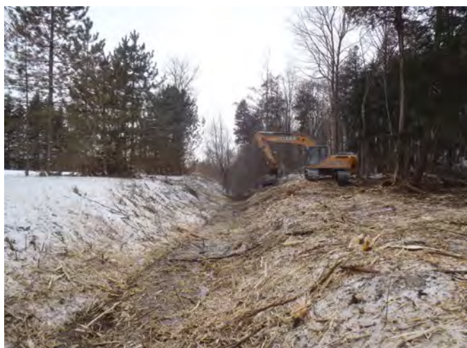
Figure A3-3. Brushing the drain bank. Source: Dietrich Engineering Ltd., Kitchener, Ontario.
