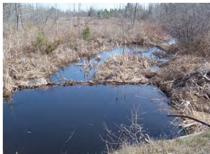
Figure B5-11. Hazeldean Road Drain – obstruction in the drain caused by beaver activity.
