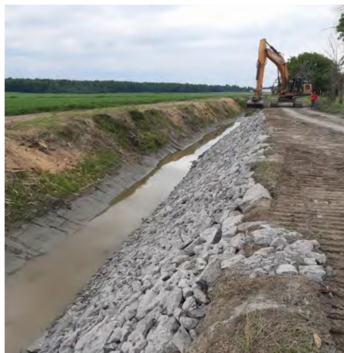
Figure B4-31. Riprap armouring of a drain. Source: Leroux Consultant, The Nation, Ontario
