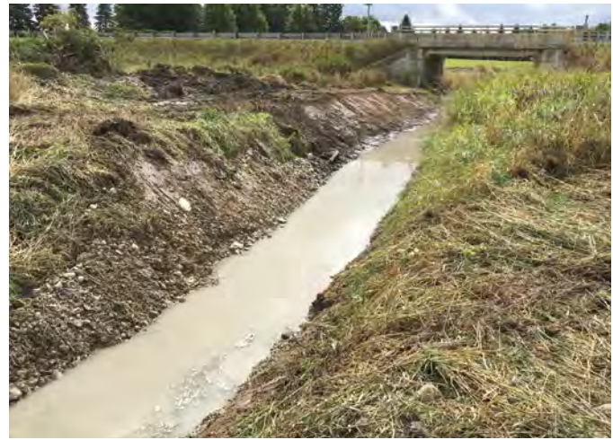
Figure A3-12. A bottom and left bank cleanout with vegetation remaining on the right bank.
