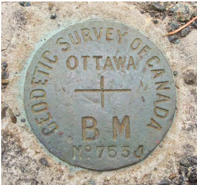
Figure A2-6. A geodetic survey benchmark.
