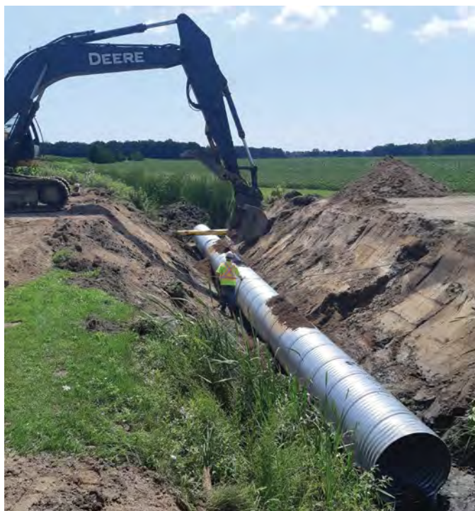
Figure A3-6. Placement of the new culvert as part of a crossing replacement.
