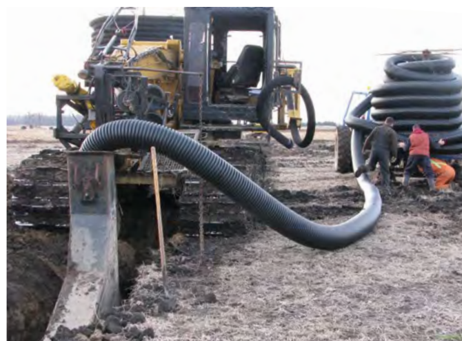
Figure A6-3. Installation of tile drainage.
