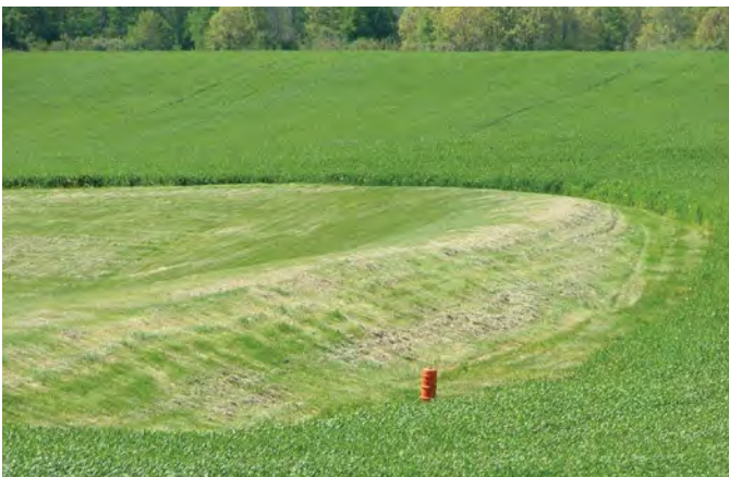
Figure B4-42. A WASCoB with berm and inlet.
