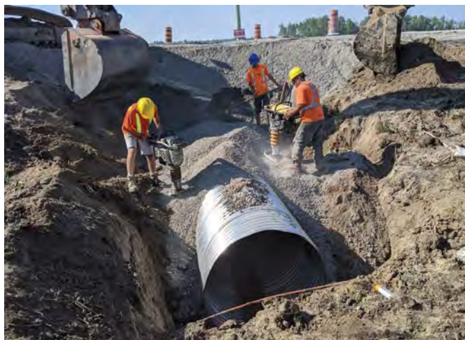
Figure A3-7. Backfilling around a new culvert.
