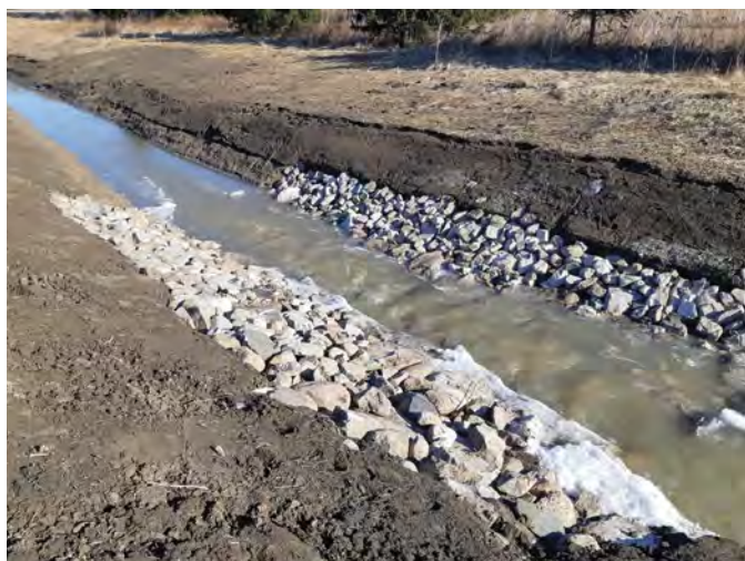
Figure B4-11. A water control structure (weir). Source: Municipality of West Elgin, Ontario
