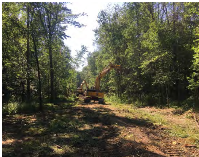
Figure A3-4. Brushing the top of a bank. Source: Dietrich Engineering Ltd., Kitchener, Ontario.
