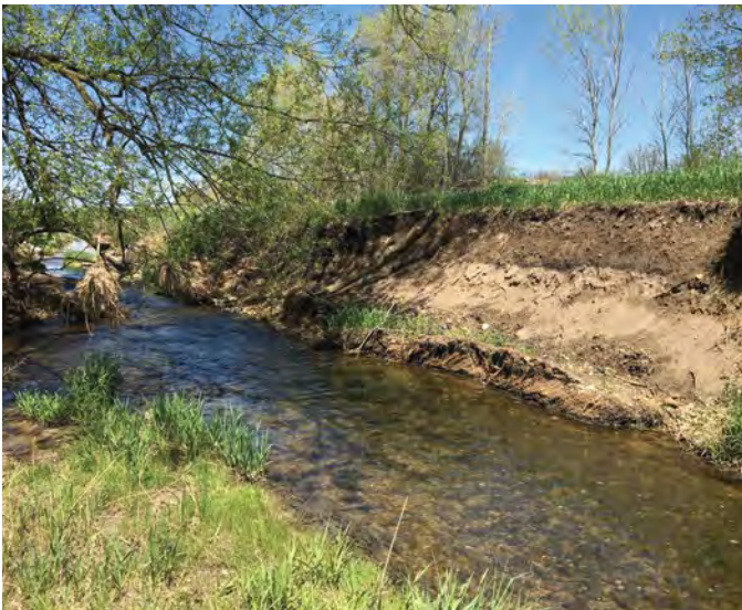
Figure B4-2. Bank failure along a drain. Source: Dietrich Engineering Ltd., Kitchener, Ontario
