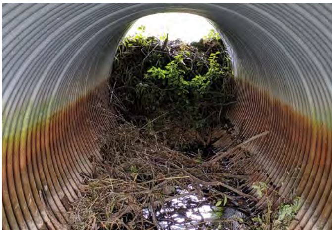
Figure A3-21. A beaver dam built on the upstream side of a culvert. Source: City of Kawartha Lakes, Ontario
