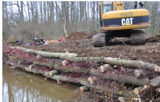
Figure B4-19. Construction of a live cribwall.
