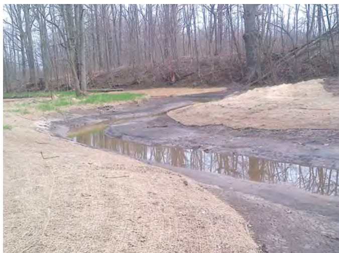
Figure B4-32. Rolled erosion control product installed on the banks of a drain.
