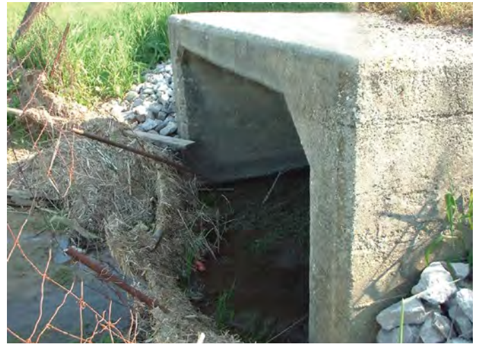
Figure A2-12. Farm fence obstructing the drain. Source: Bill Mayes, Norfolk County, Ontario
