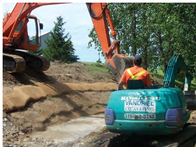
Figure B5-10. Steenstra Drain – Construction of the bioengineered channel bank. Source: Municipality of Central Huron, Ontario
