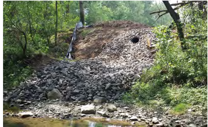
Figure A3-8. Bank stabilization and outlet repair. Source: Leroux Consultant, Municipality of Champlain, Ontario
